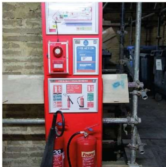
An example of a good fire point on site
